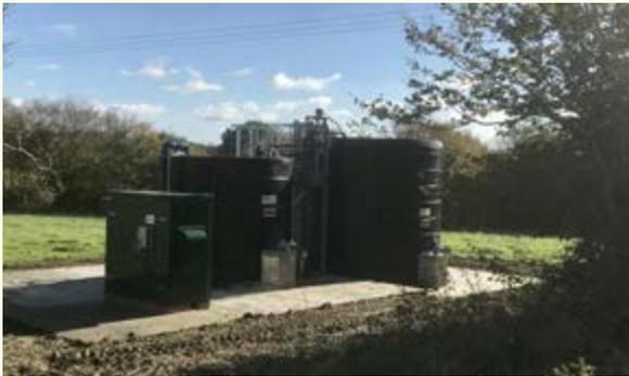
Two tanks are needed - first a balance tank into which all winery waste water, solids and domestic effluent is drained and second, a reactor tank where the bulk of the treatment takes place. Bacteria which break down the solid matter are introduced making it clean enough to be released into the water table.
